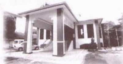
Penang First Assembly of God 286, Macalister Road, 10450 Penang, Malaysia
